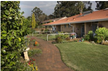
The new units
